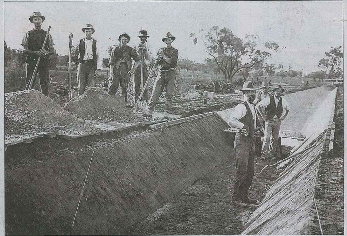
In times gone by: at Merbein, irrigation water was initially delivered in channels and distributed to plants in furrows.
